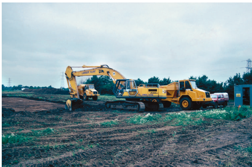
Plate 1.2 Lake End Road West stripping the topsoil
